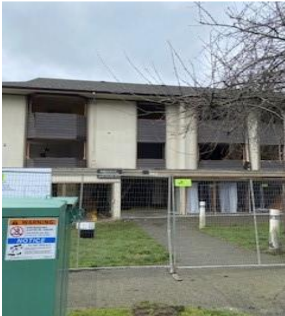
Newbridge prep for demolition
