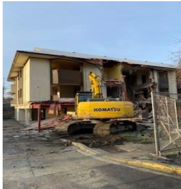
Start of Newbridge demolition
